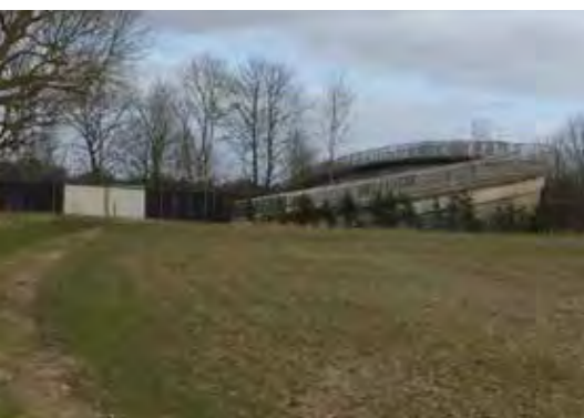
Cantelope Farm - M11 bridge
