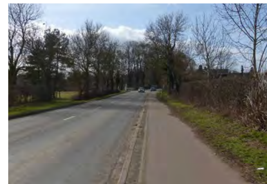
Existing photograph of the Burwash Manor entrance
