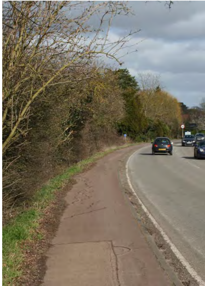
Shared footway/cycle path along Barton Road - outside the City
