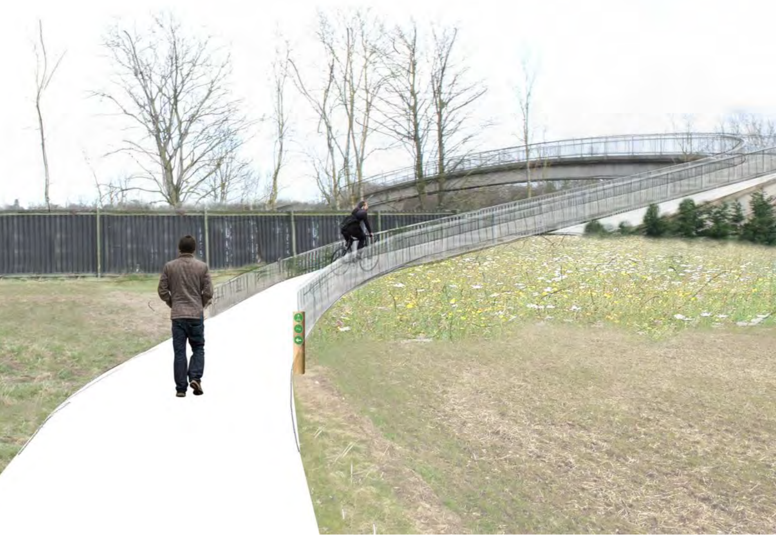
Ha.7.A - Cantelope Farm - M11 bridge
