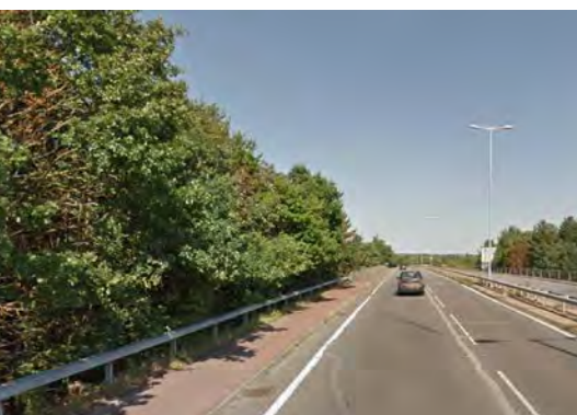
Existing photograph of Barton Road - bridge over M11
